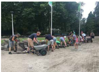
Workshop Pile Walls at the Entrance Area
